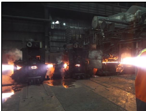
Figure 2.2. Rolling mill in ArcelorMittal Zenica
