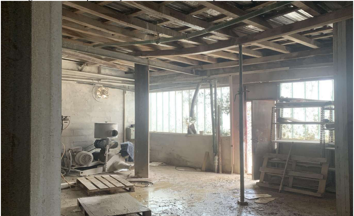
Figure 8. Detailed position of the wooden and steel section supports to plastically deformed sections
