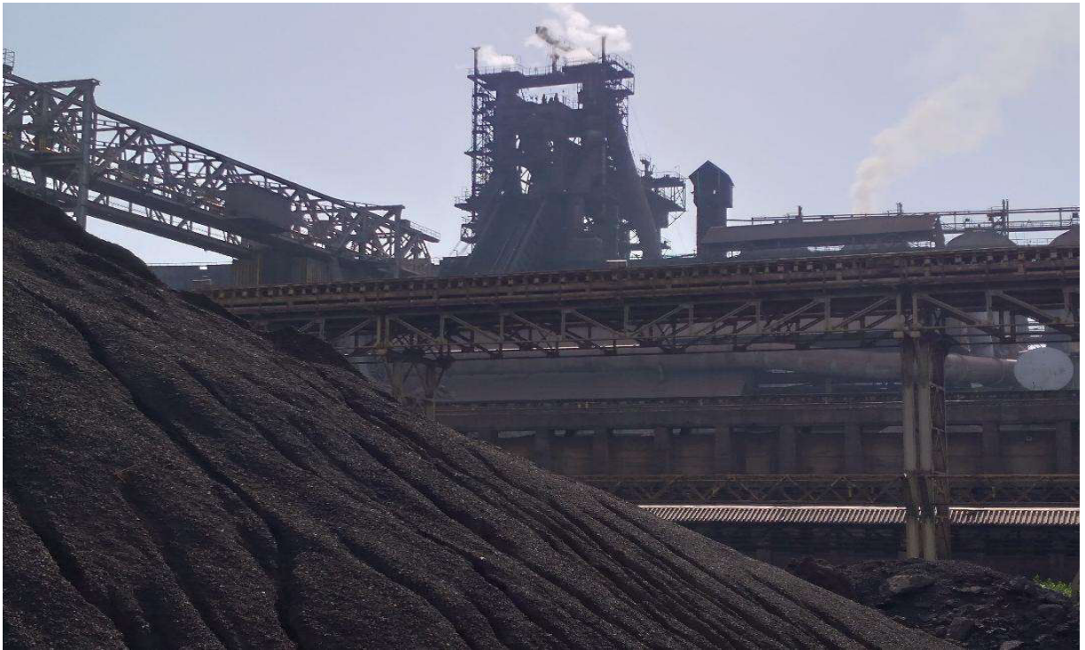
Figure 3. Eastern layout view from a broken portal crane
