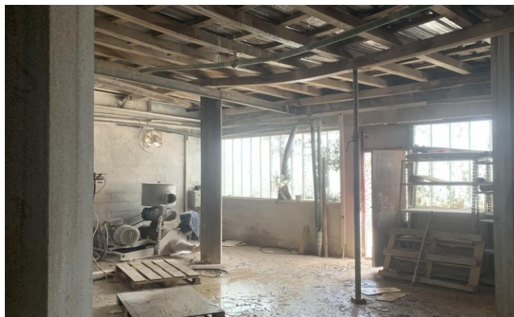
Figure 10. Another location of the wooden and steel construction supports to plastically deformed sections
