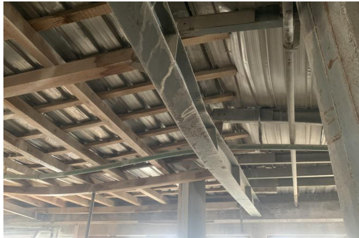
Figure 9. Position of the wooden and steel construction supports to plastically deformed sections
