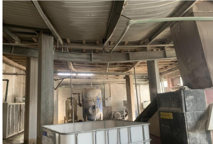
Figure 12. Detailed position of plastically deformed sections & roof
