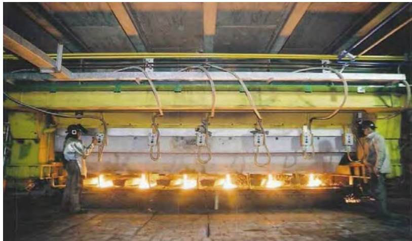
Figure 1. Tundish with a capacity of 35 tonnes with six strands.
