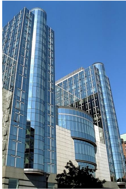
Figure 6. Altieri Spinelli Building, Brussels, Belgium [20]
